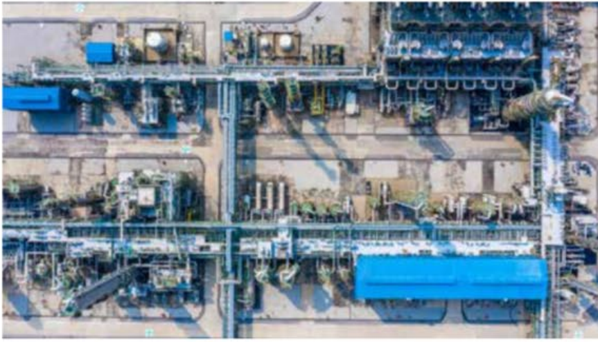
Figure 1. Aerial view of a hydrogen plant at a refinery.
