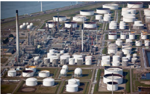
Figure 2. Refineries and tank farms require flammable and toxic gas detection.
