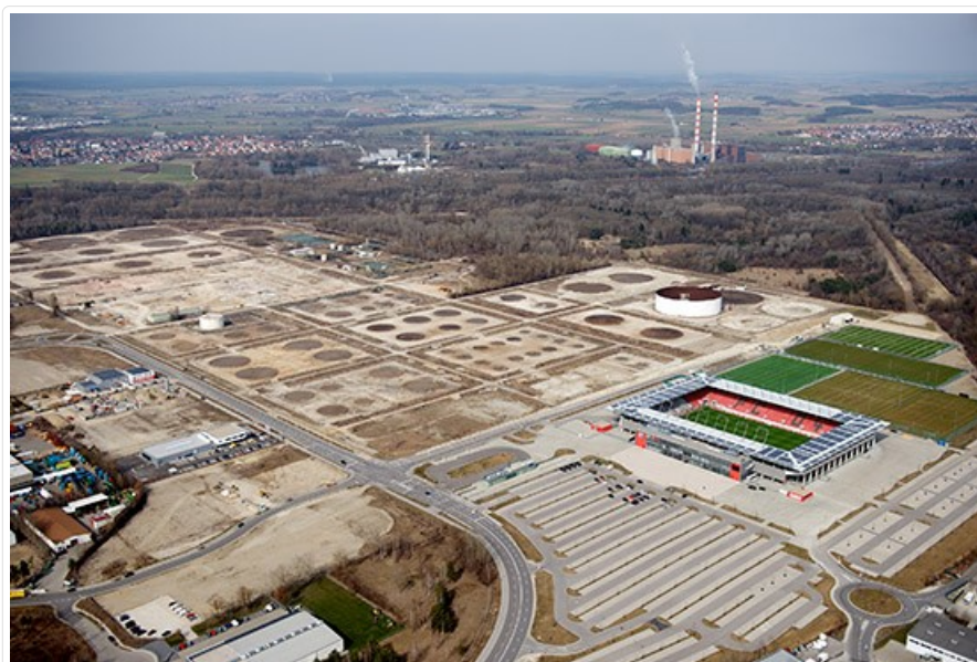
Refinery decommissioning in April 2013 (copyright Bayernoil Raffineriegesellschaft GmbH).
