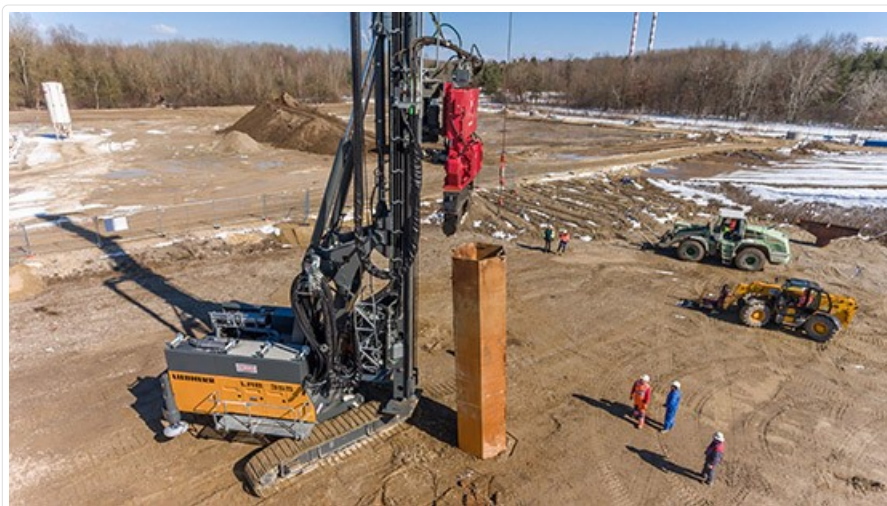
IN-Campus Pile driving for ground water capture (copyright AUDI AG).
