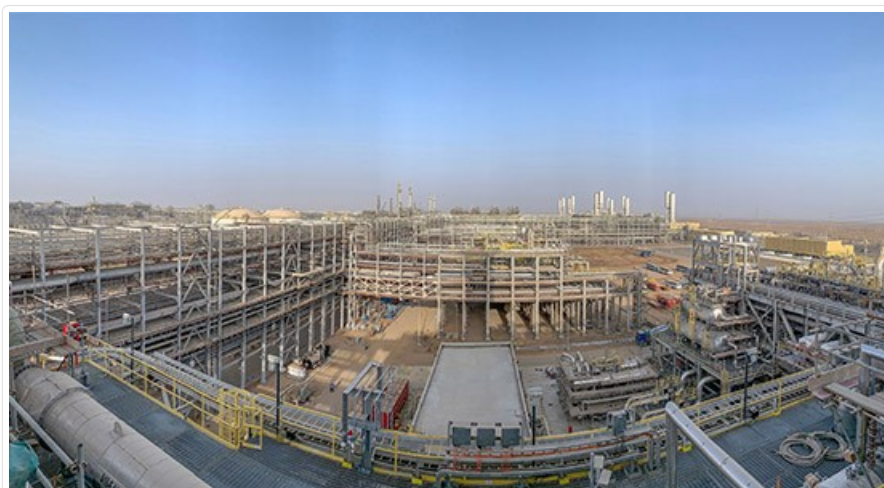
Jazan refinery and integrated gasification combined cycle power plant under construction.
