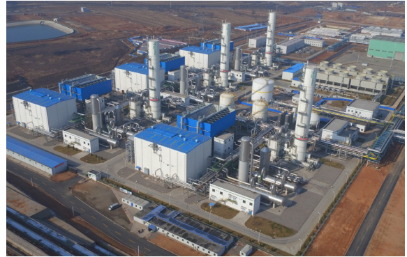
Image courtesy of Air Products and Chemicals Inc. Four ASUs to feed the gasifiers at Lu'an
