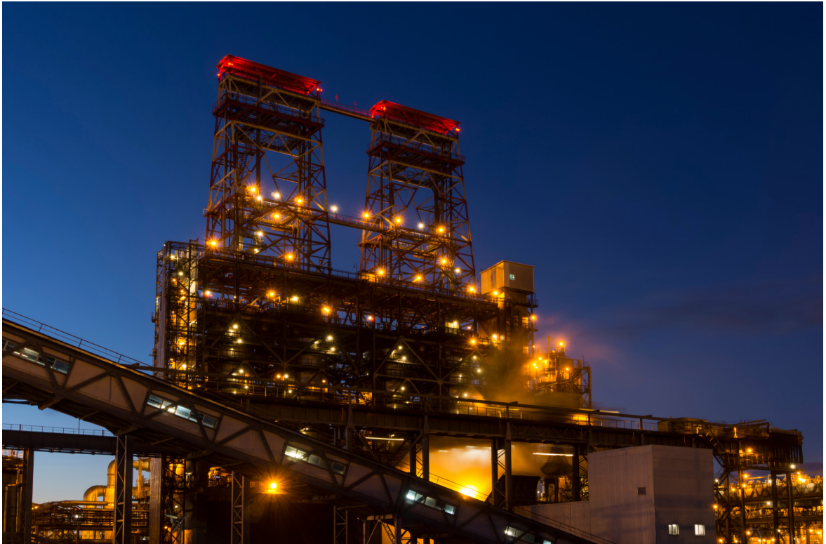
Four drum delayed coker unit
