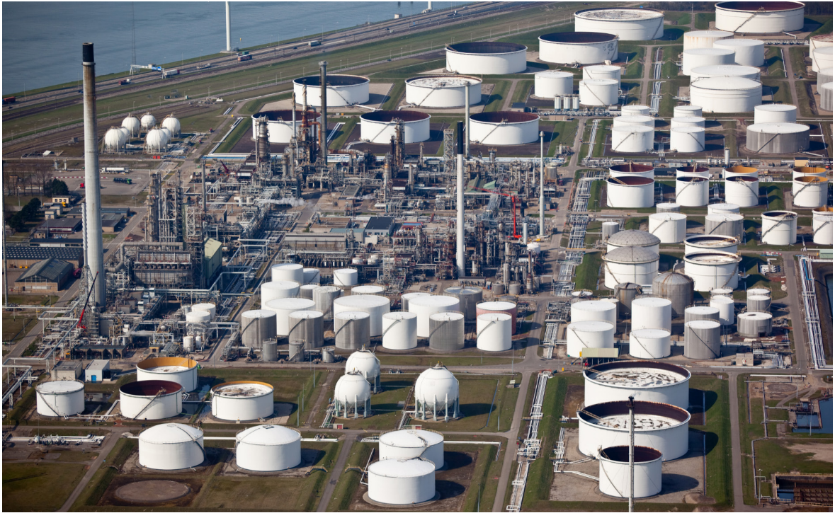
Oil refinery with refined products storage
