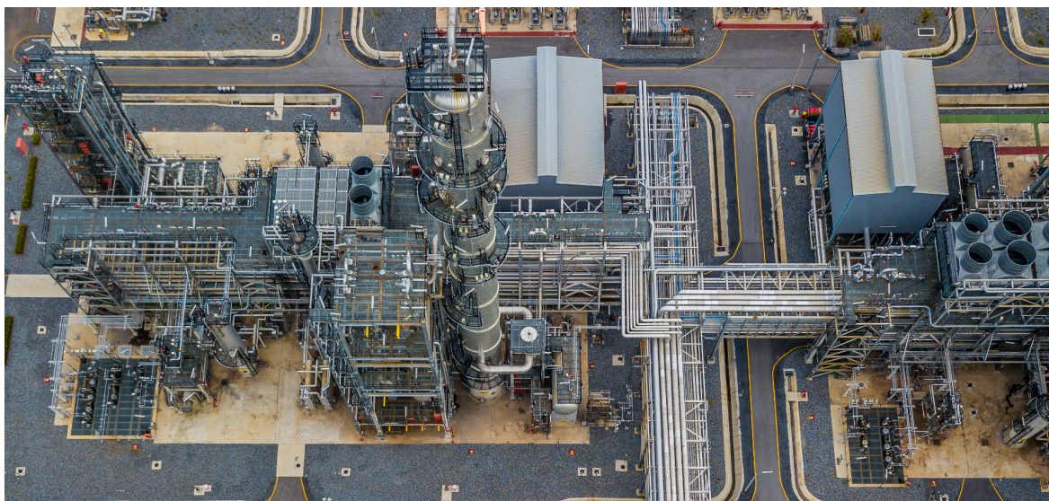
SMR for refinery hydrogen production
