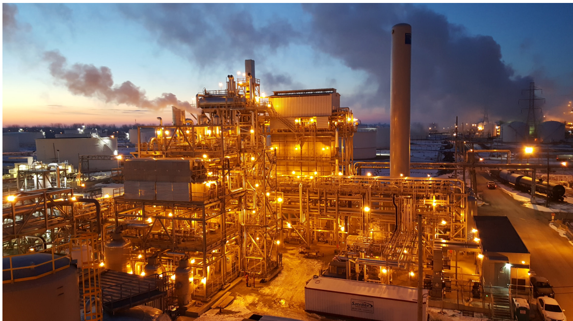
SMR at Lima, Ohio - image courtesy of Matheson Tri-Gas Inc
