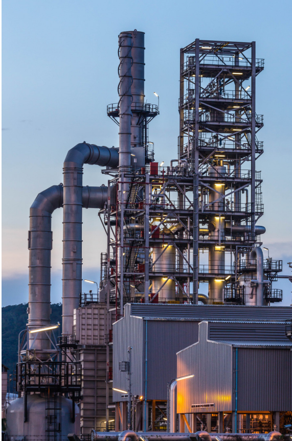
Refinery hydrogen production on a Steam Methane Reformer
