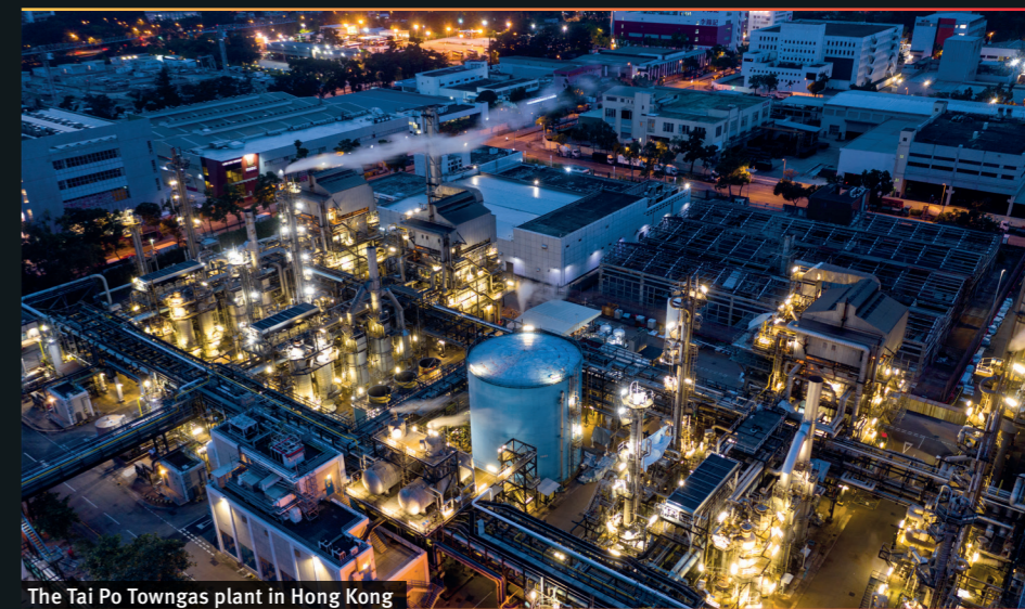
The Tai Po Towngas plant in Hong Kong
