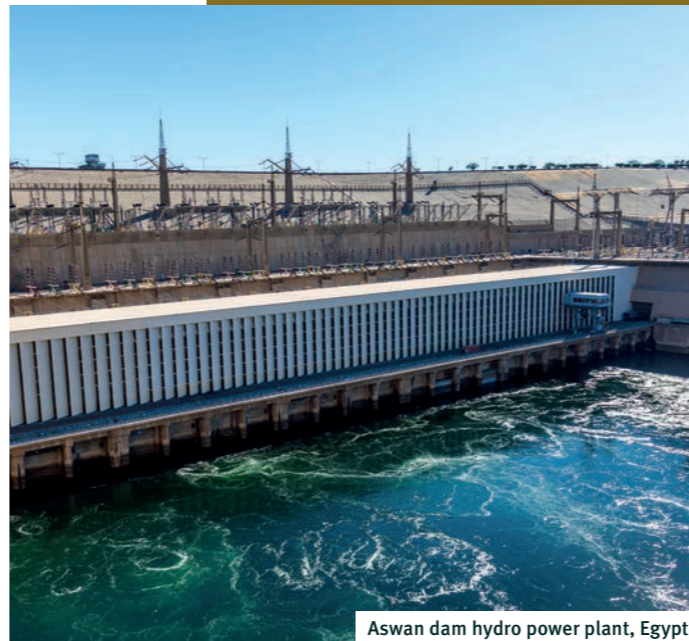
Aswan dam hydro power plant, Egypt.
