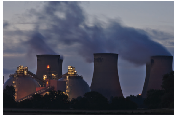
DRAX Power Station UK
