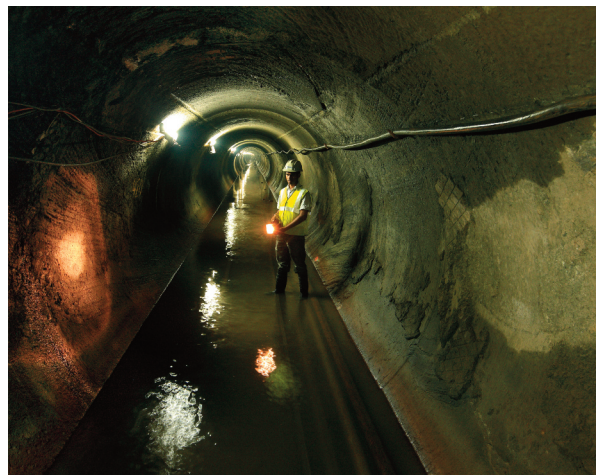
Part of a sewer network in Mumbai, India
