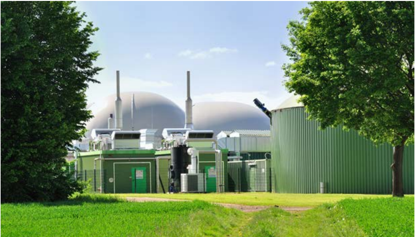
Biogas plant with biomethane upgrade and CHP units
