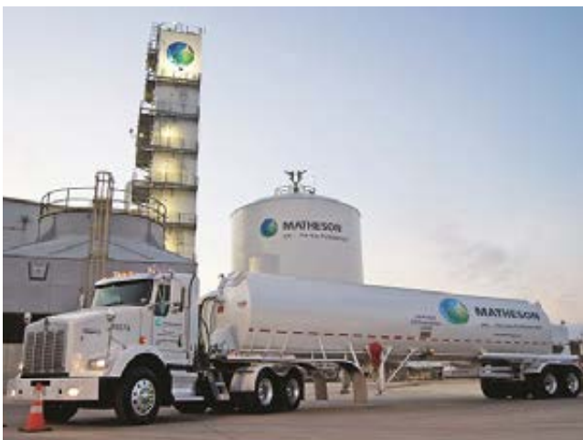
A merchant ASU for the production of liquified oxygen, nitrogen and argon. Copyright Matheson Tri-Gas Inc.
