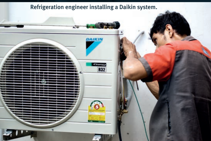
Refrigeration engineer installing a Daikin system.
