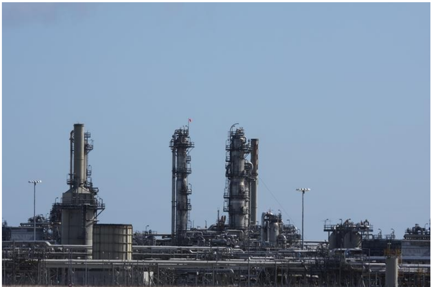
St Fergus gas terminal, north of Aberdeen
