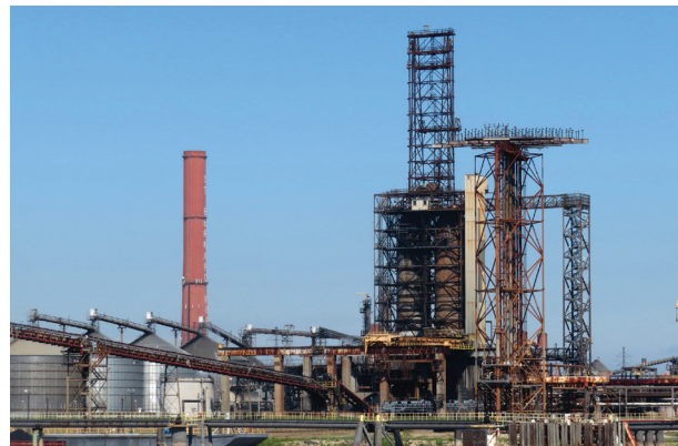
Delayed Coker on a refinery
