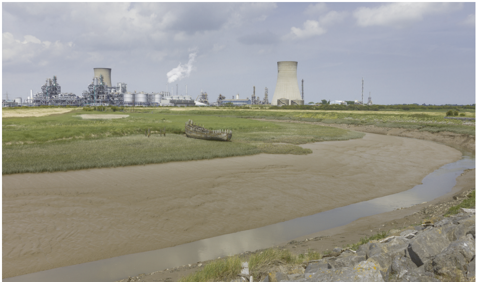
Saltend Chemicals Park on the North bank of the Humber River. Equinor’s H2H Saltend project will produce blue hydrogen by reforming natural gas whilst capturing its CO 2 emissions, which will be stored under the North Sea
