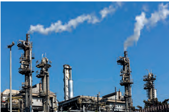
Hong Kong Town gas production with reforming of hydrocarbons to syngas
