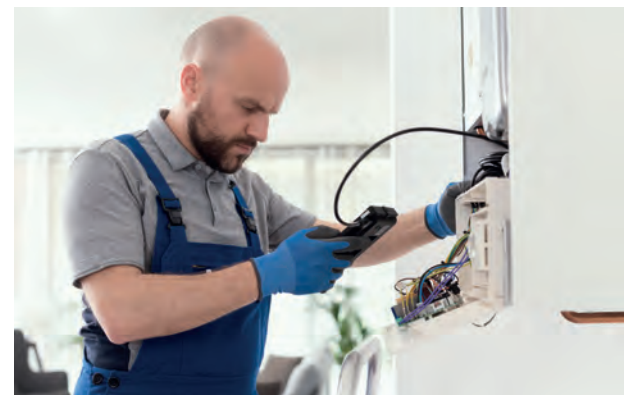
Testing flue gases from a domestic boiler
