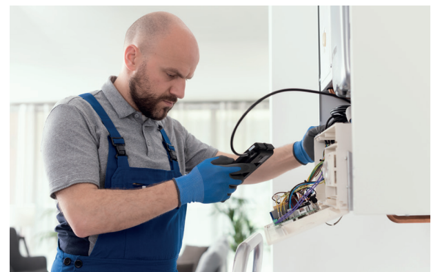
Testing flue gases from a domestic boiler
