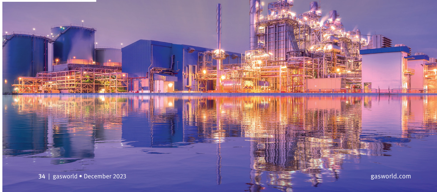
Gas-fired power plant
